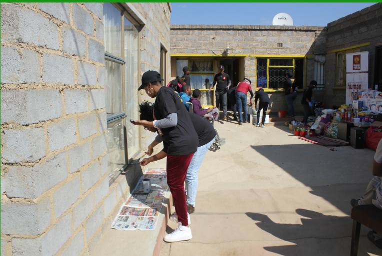
Karabo Kgasago and Delia Malahlela painting the window frames.
